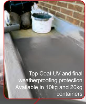
**Top Coat UV and final weatherproofing protection**
