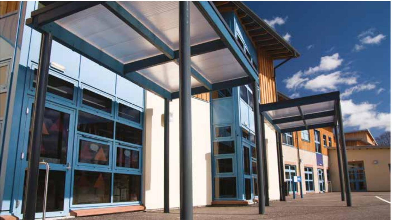
Marlon Clickfix RL is a glazing system suitable for use in pitched rooflights, northlights and canopies. The glazing system combines perfectly with the click and fix mechanism of the Marlon Clickfix1040 multiwall polycarbonate glazing panels for seamlessly glazed rooflights with no visible fixings.
