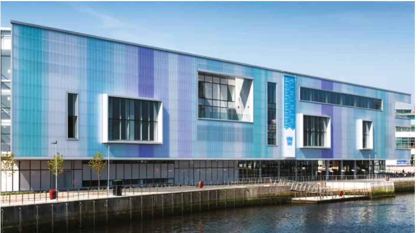
Designed for vertical glazing applications, Marlon Clickfix VF is the ideal solution for seamlessly glazed facades, partitions and cladding, internally and externally. Glazed with Marlon Clickfix1040 polycarbonate panels, installation is straightforward as the glazing simply clicks and fixes into place to create uninterrupted light walls of unlimited size and shape.
