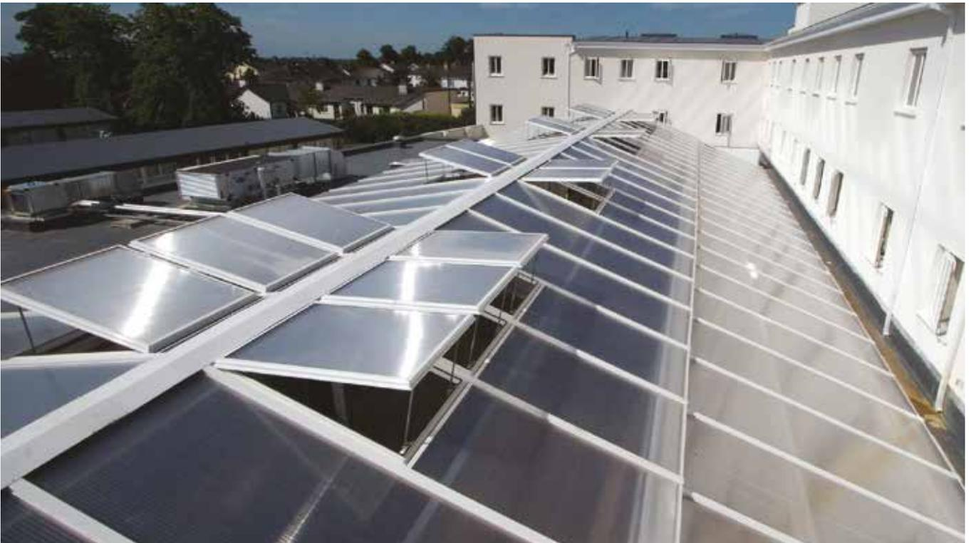
Xlok Ultra is a 'fast fit' panel glazing system consisting of panels which simply link together on site for quick installation and runs of unlimited length.
