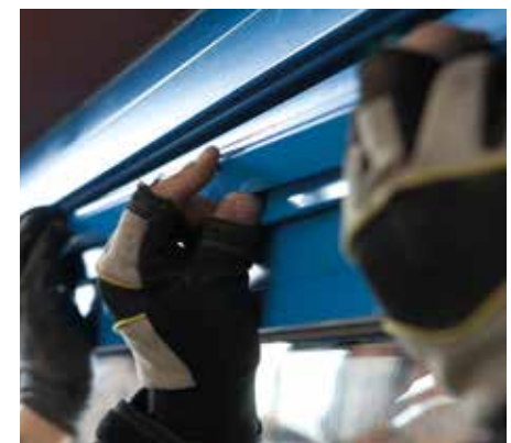
Framing clips and seals secure the window in place. These sections can be removed to allow replacement of the glazing element.
