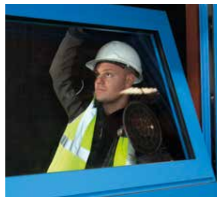
The window can be fitted from the inside at a later date, providing flexibility and time savings to the build program.
