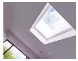
Featuring an ultra-modern flat glass design, Mardome Glass is a thermally efficient double glazed rooflight incorporating a silver anodized aluminium frame (with the option to powder coat), which combines to deliver high end design and the very best standards in security and safety.
