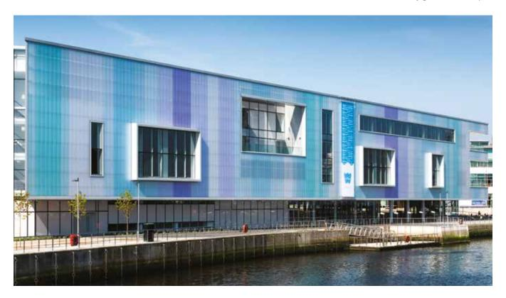
Designed for vertical glazing applications, Marlon Clickfix VF is the ideal solution for seamlessly glazed facades, partitions and cladding, internally and externally. Glazed with Marlon Clickfix1040 polycarbonate panels, installation is straightforward as the glazing simply clicks and fixes into place to create uninterrupted light walls of unlimited size and shape.
