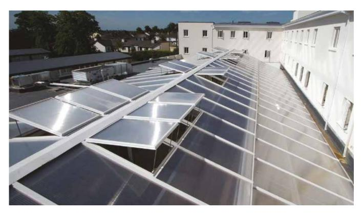
Xlok Ultra is a 'fast fit' panel glazing system consisting of panels which simply link together on site for quick installation and runs of unlimited length.
